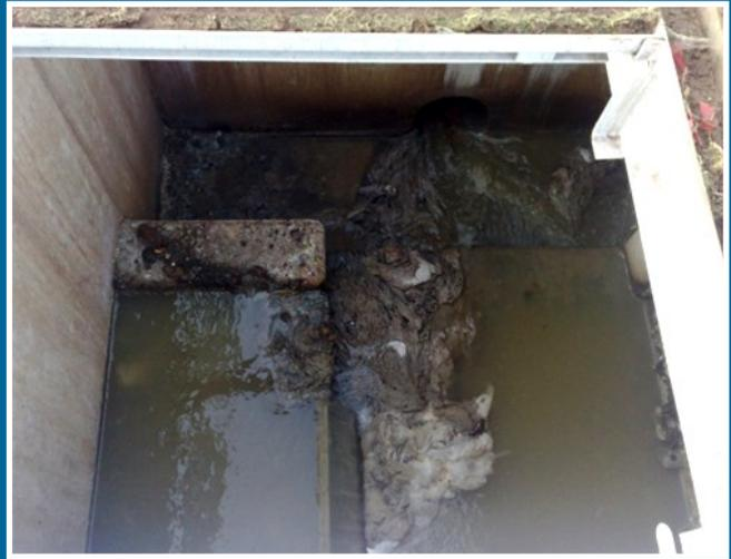
**Figure 1: CSO spilling litter due to blocked screen**
